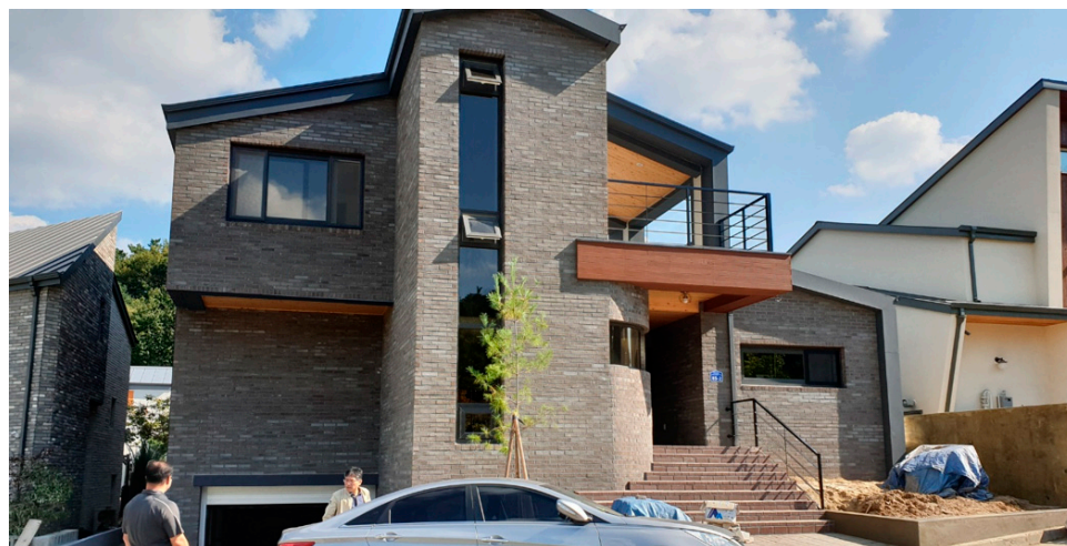
Figure 1. Overview of the residential building equipped with energy slabs.
