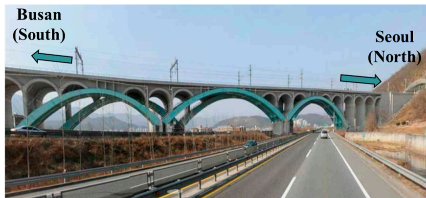
Figure 1. Eonyang Arch Bridge.
